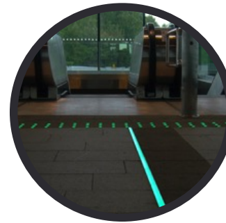
Floor tactile signage
