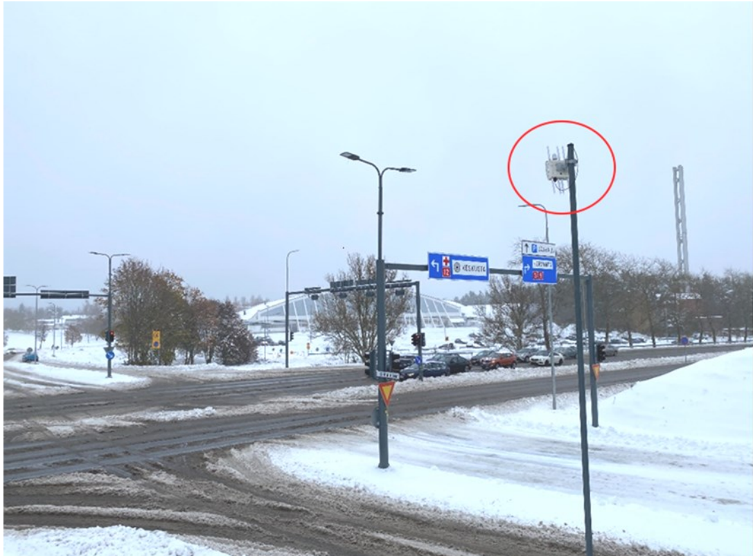
Figure 7. RSU installation at the intersection
